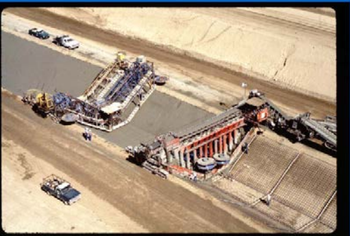
Paving canal liner
