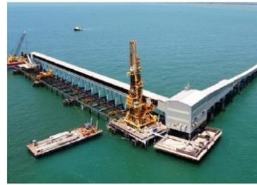
*Figure 4 Bulk export terminal used to load sugar onto ships for export*
